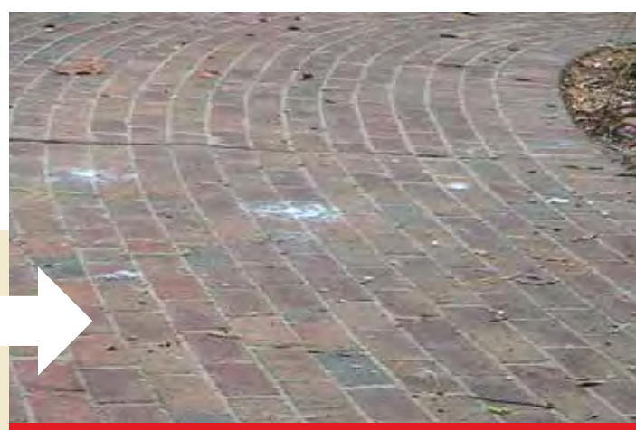
After (Like new with no costly excavation)
