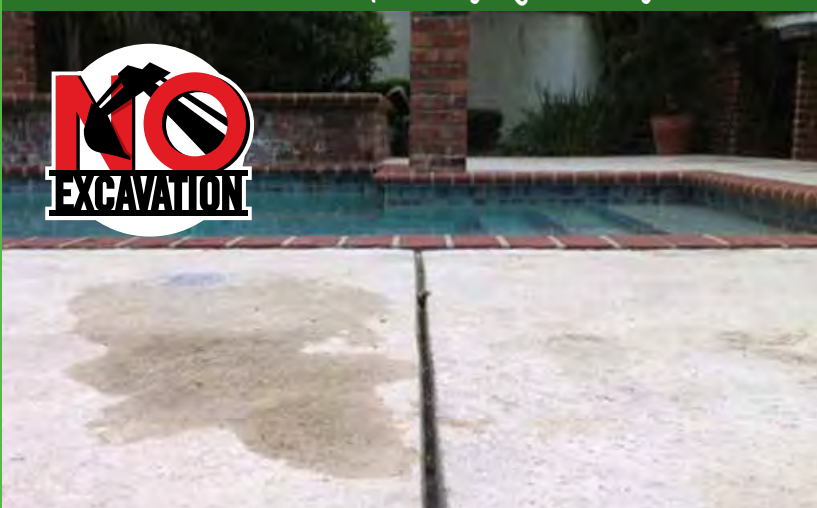
After (Just like new with no excavation!)
