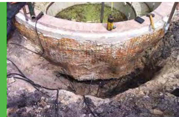
Before (Spa dropped 4.5" from original elevation)
